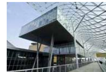
MILAN EXHIBITION CENTRE N. 330 AHU - 11.000.000 m 3 /h Rho (IT)
